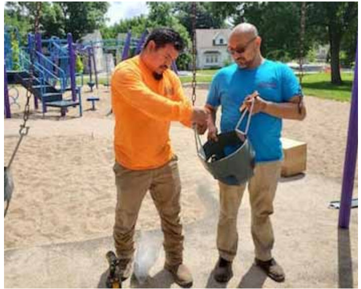
Francisco and Solomon of FJC Builders installing the new seats...
